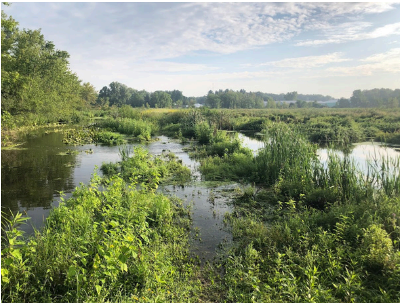
Kline Levee water control structure during a flood event, July 2024
